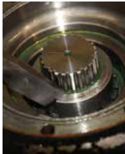
5. Remove lock nut using a chisel and hammer
