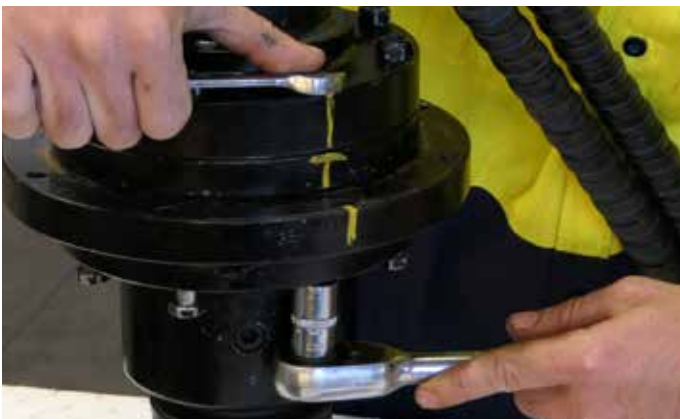
27. Replace the motor and motor bolts lining up previously marked alignment lines (Loctite 243 Thread locker - medium strength on bolts). PDD: Motor bolts not applicable.
